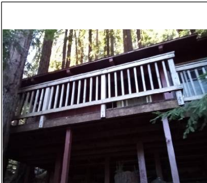
Deck at cabin 9.
