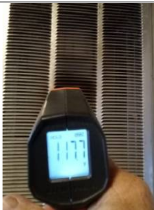
Temperature at wall furnace.
