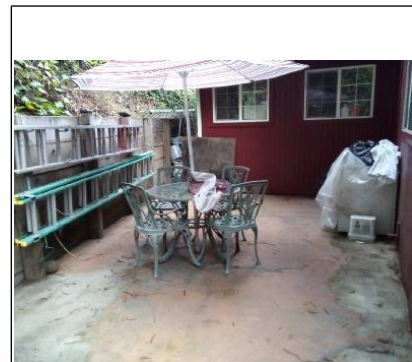
Patio at rear of house was found to be in satisfactory condition at time of inspection.
