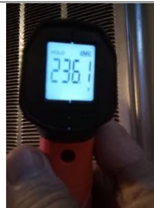
Temperature at wall furnace.
