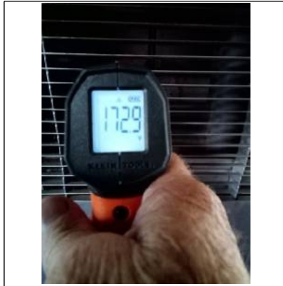
Temperature at wall furnace.
