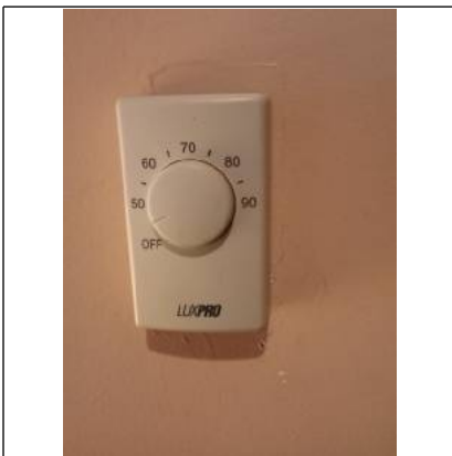
Thermostat present no baseboard heater was discovered in room.
